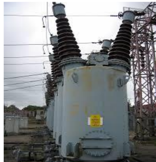
Fig.2.3 Bulk oil circuit breaker
