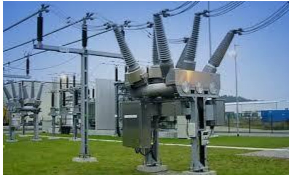
Fig.2.4 Minimum oil breakers
