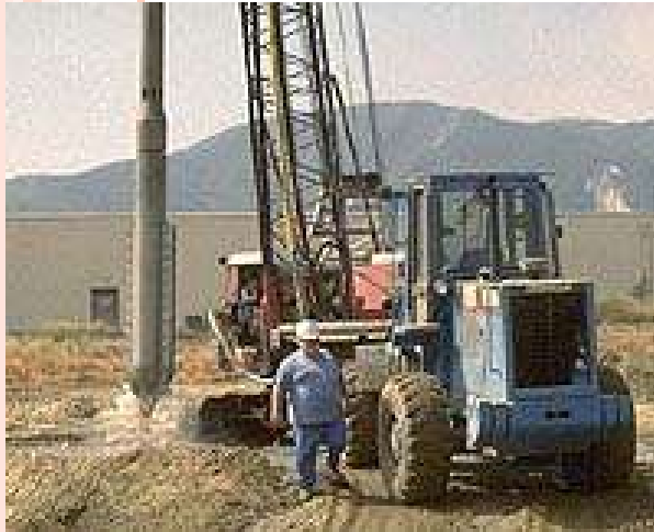
Top-feed vibroflot rig
