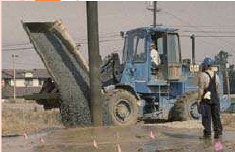
Adding stone in top-feed installation
