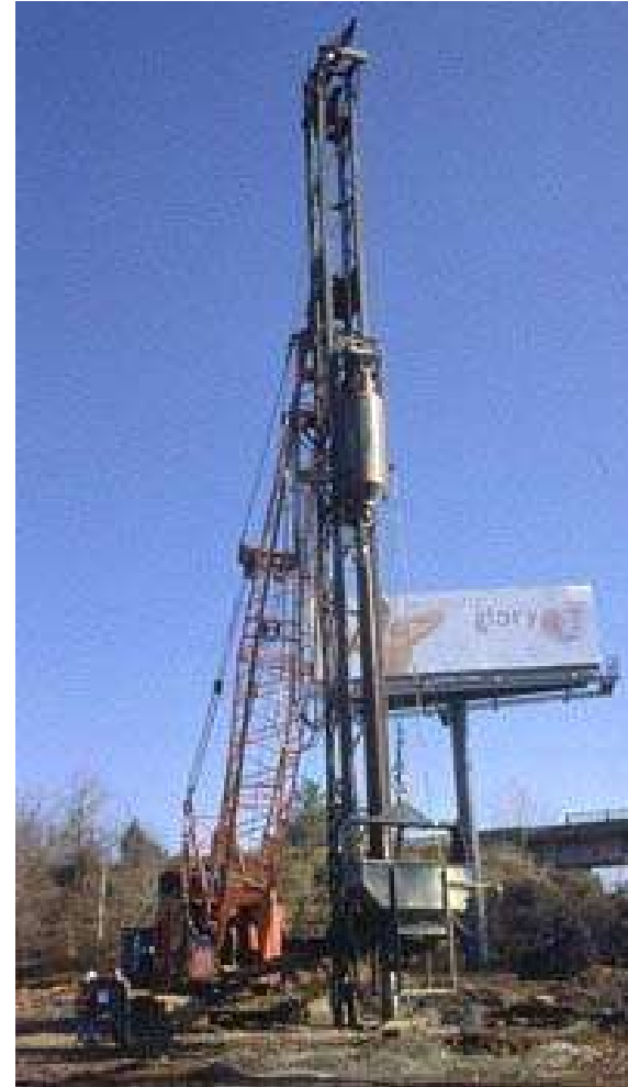
Bottom-feed vibroflot rig
