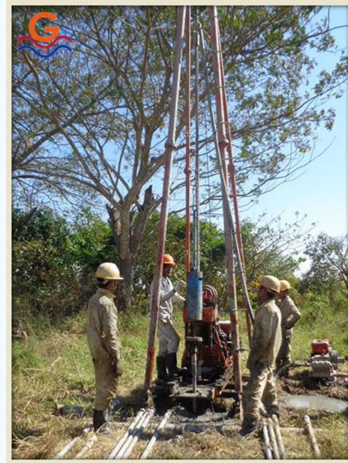
Standard penetration test (SPT)
