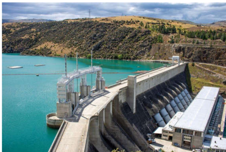
Hydraulic power station
